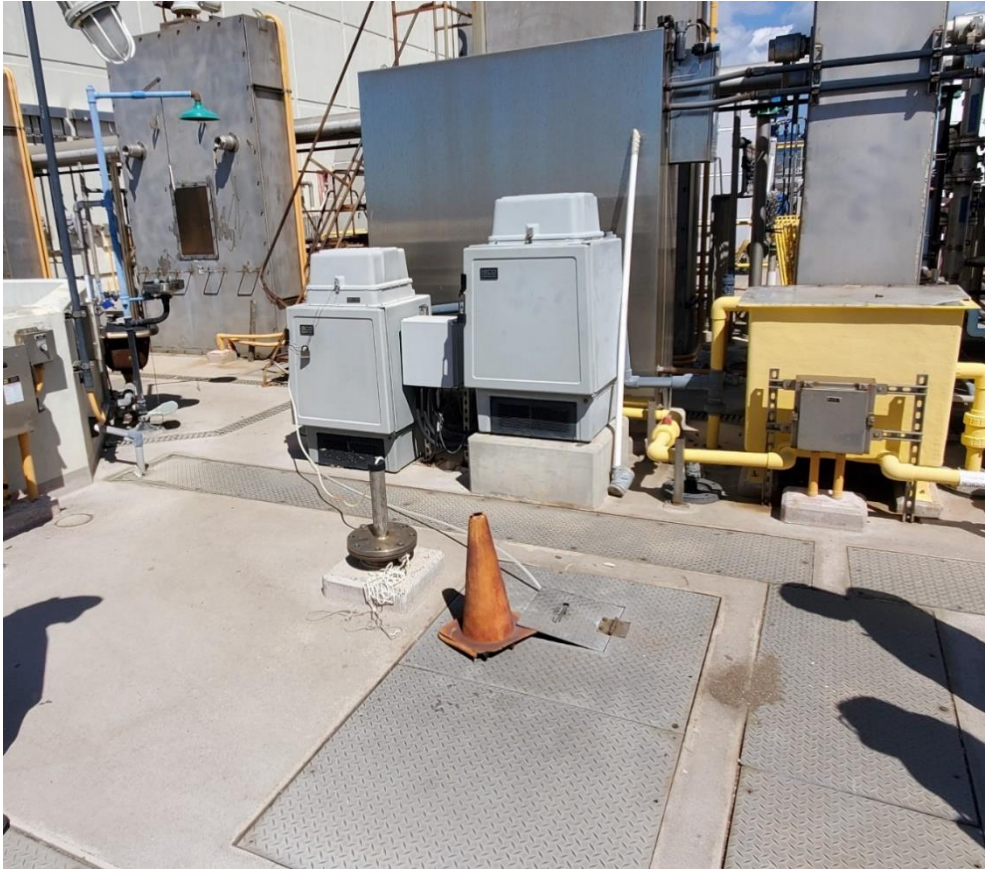
Sand Island WWTP Influent Sample Point
